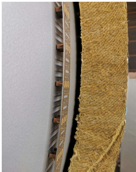
Figure 5 - ESSGE NCS Spacer Band around a large tank with polymer legs facing inward.
