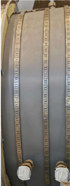
Figure 2: ESSGE NCS band on a large tank with maximum 400mm spacing
